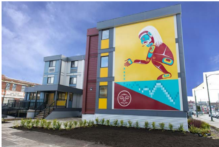
Figure 8: Photo of 220 Terminal Avenue, Canada
