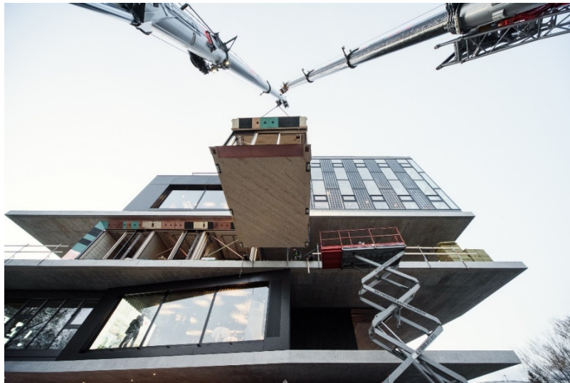
Figure 14: Installation of the UMAR Unit to the Nest Research Building
