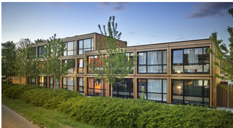
Figure 12: Photo of the Project in Leiden with the Finch Buildings System https://circulairebouweconomie.nl/wp-content/uploads/2022/01/Circular-Buildings-Strategies-and-case-studies-2021.pdf , accessed Oct 2024.
